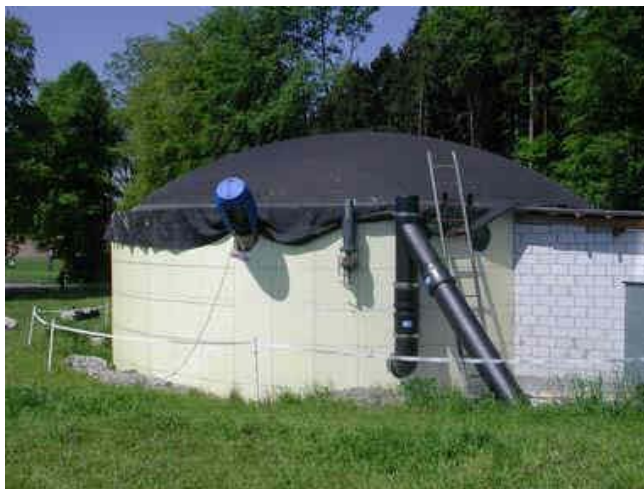
Installation de biogaz
